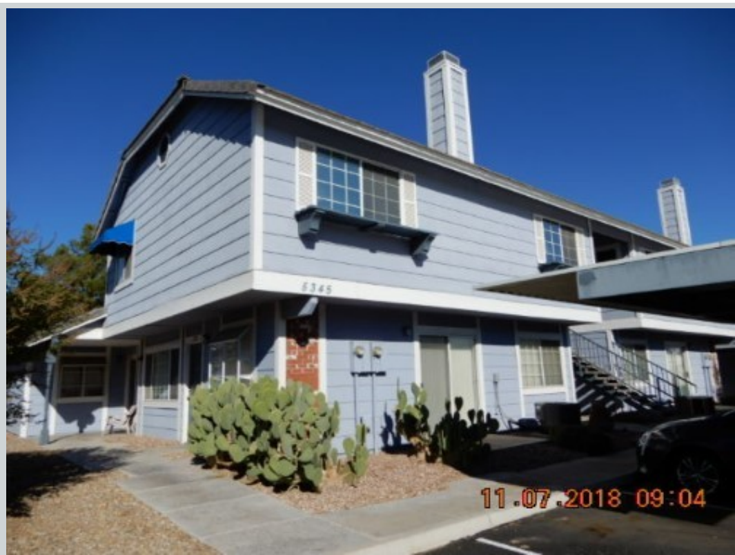
Subject 5345 Silvermist Ct Unit 202 View Front Comment "Front of building."
