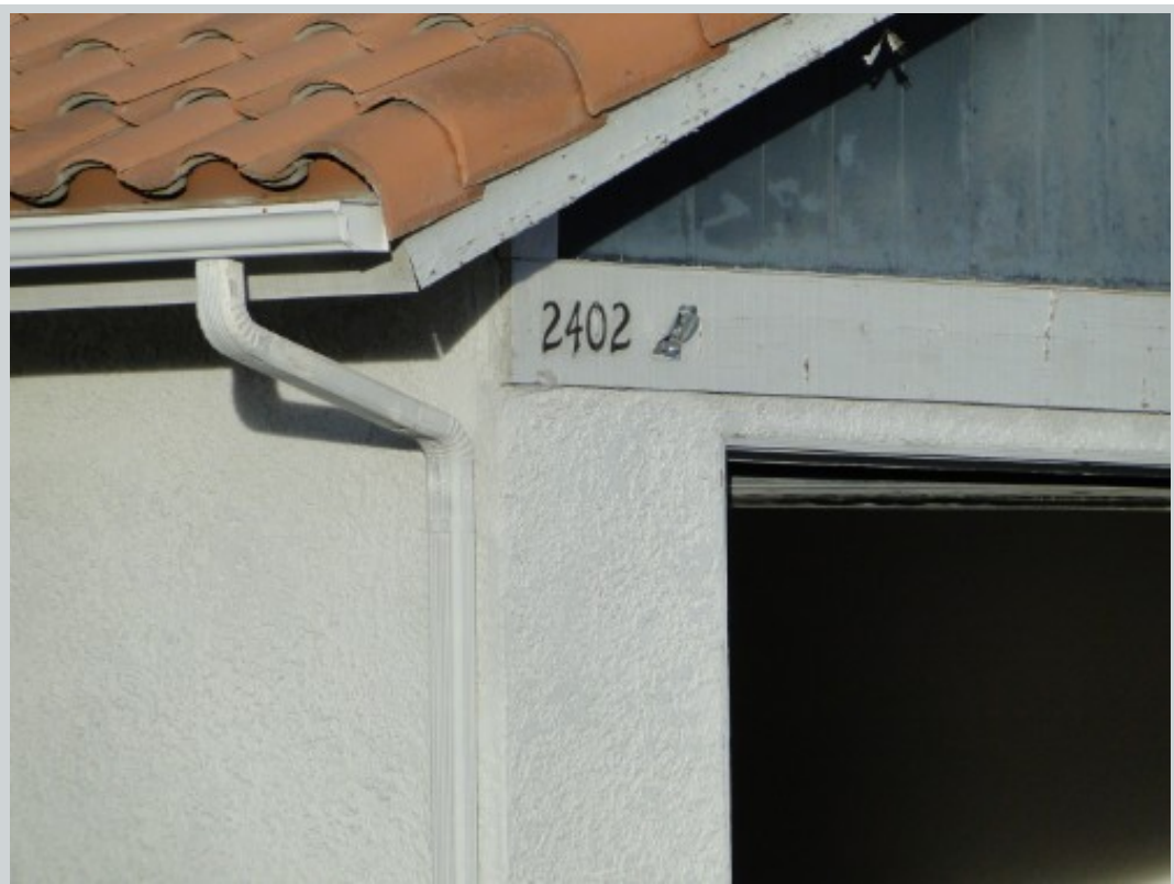
Subject 2402 Muirfield Ave
