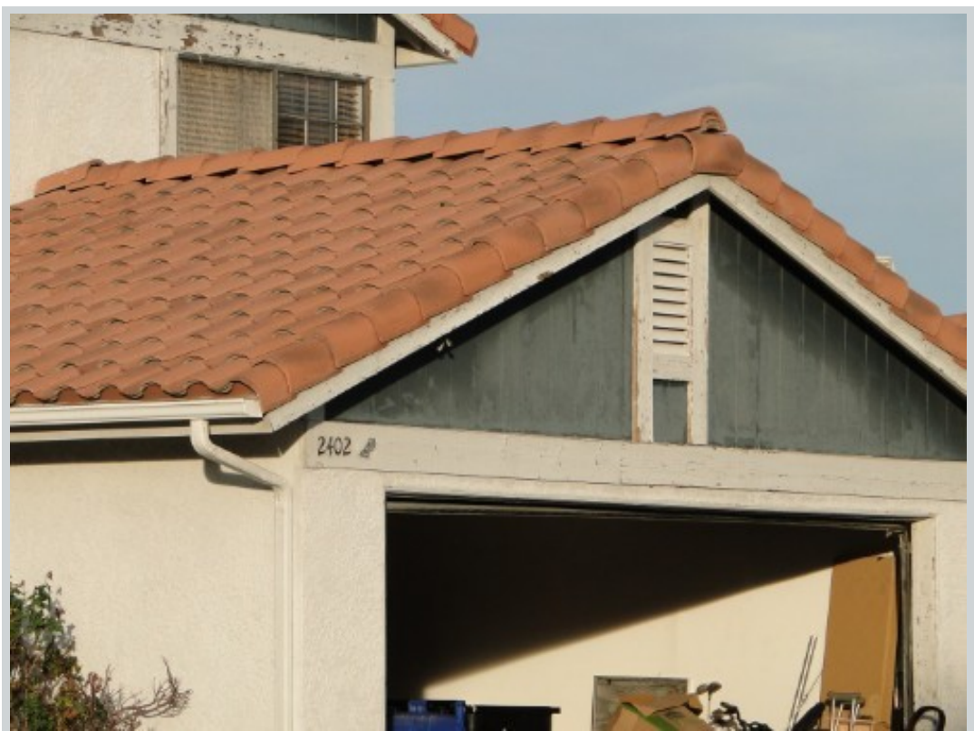
Subject 2402 Muirfield Ave
