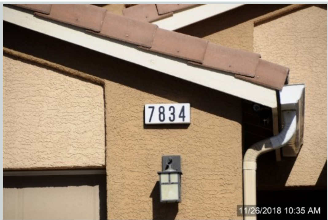
Subject 7834 Whitlocks Mill Ave
