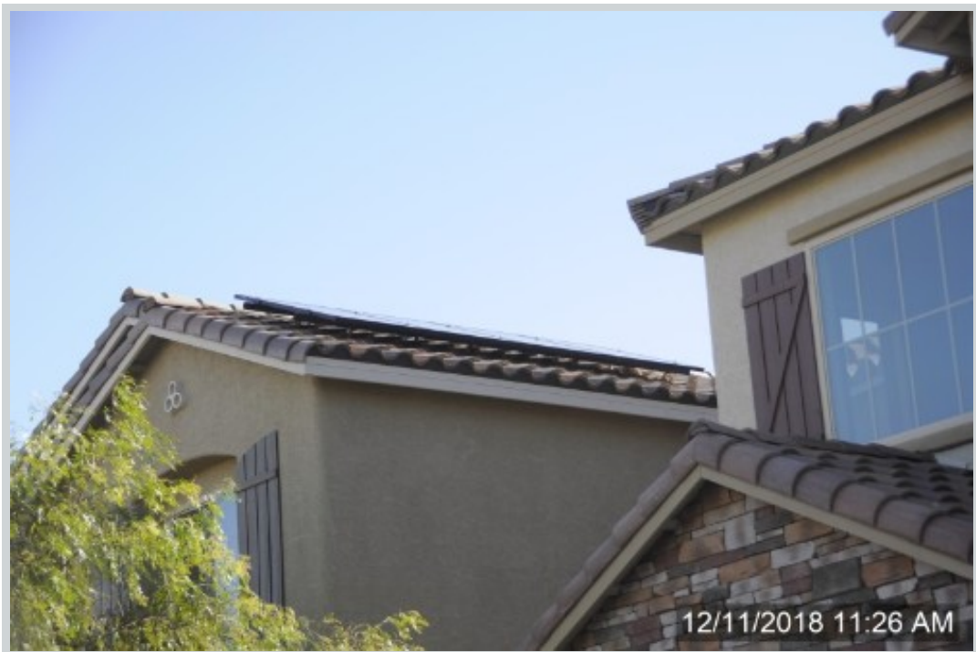
Subject 10651 Harley Cross Ct View Other Comment "Solar Panels on the Subject's Roof, Unknown Ownership"
