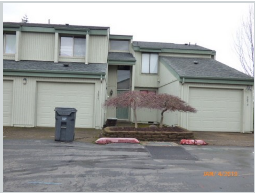
Subject 3877 Auburn Rd Ne
