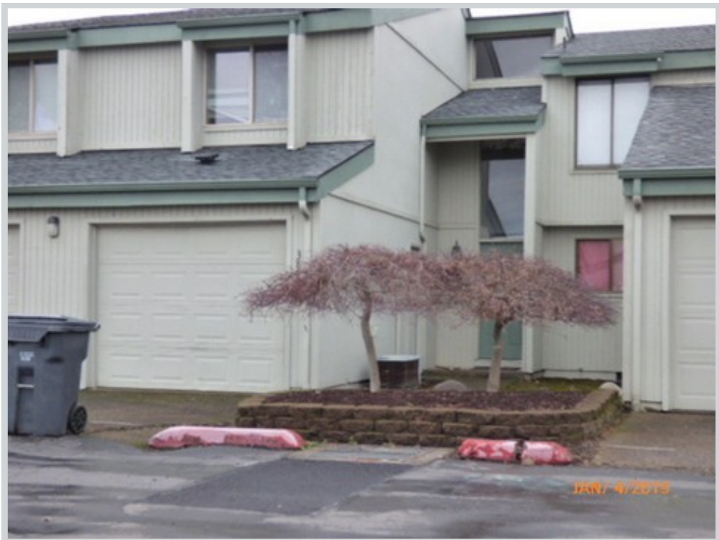
Subject 3877 Auburn Rd Ne
