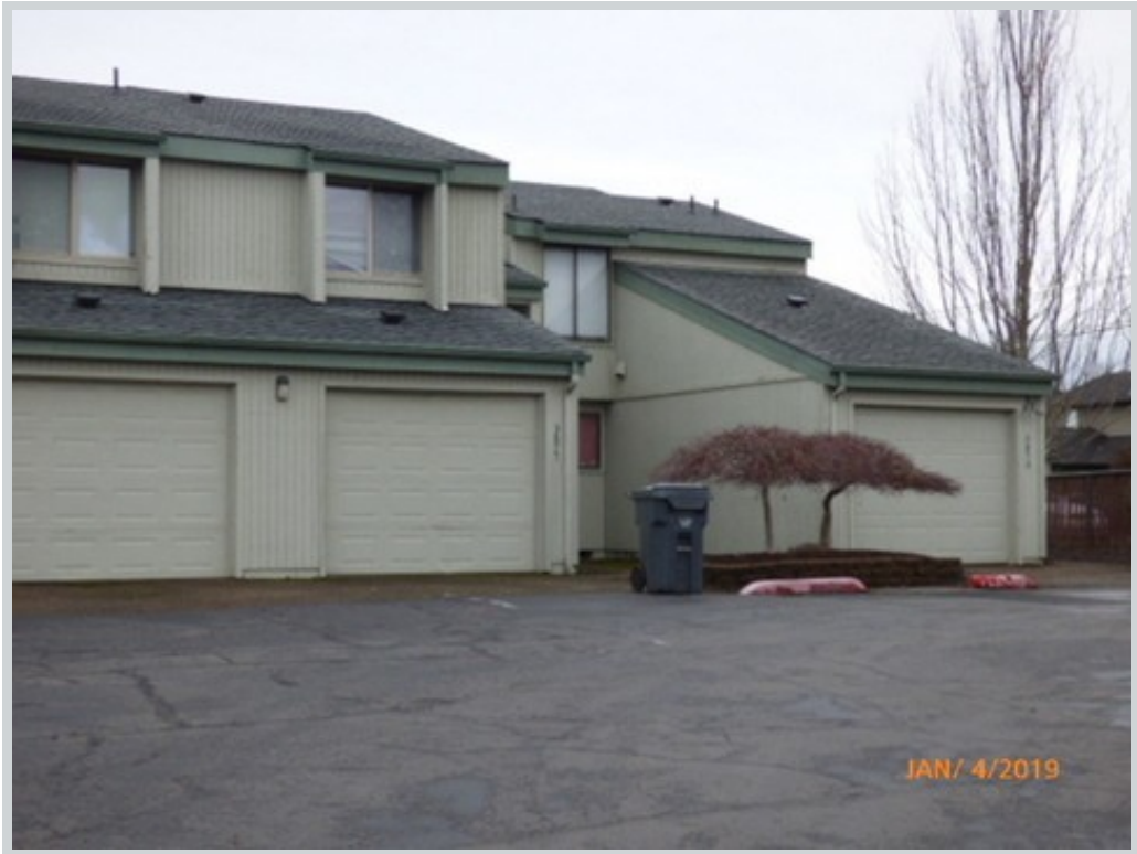
Subject 3877 Auburn Rd Ne
