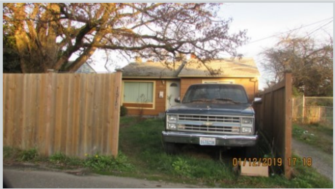
Subject 1515 S Trafton St
