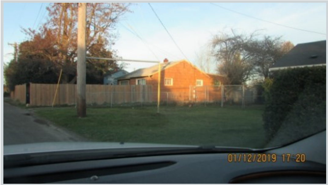
Subject 1515 S Trafton St
