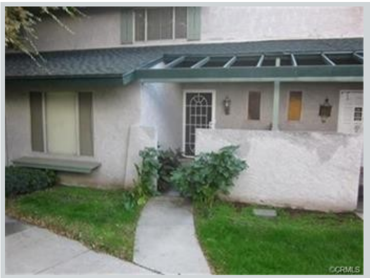
Listing Comp 1 3600 Mountain Ave Apt 20f View Front
