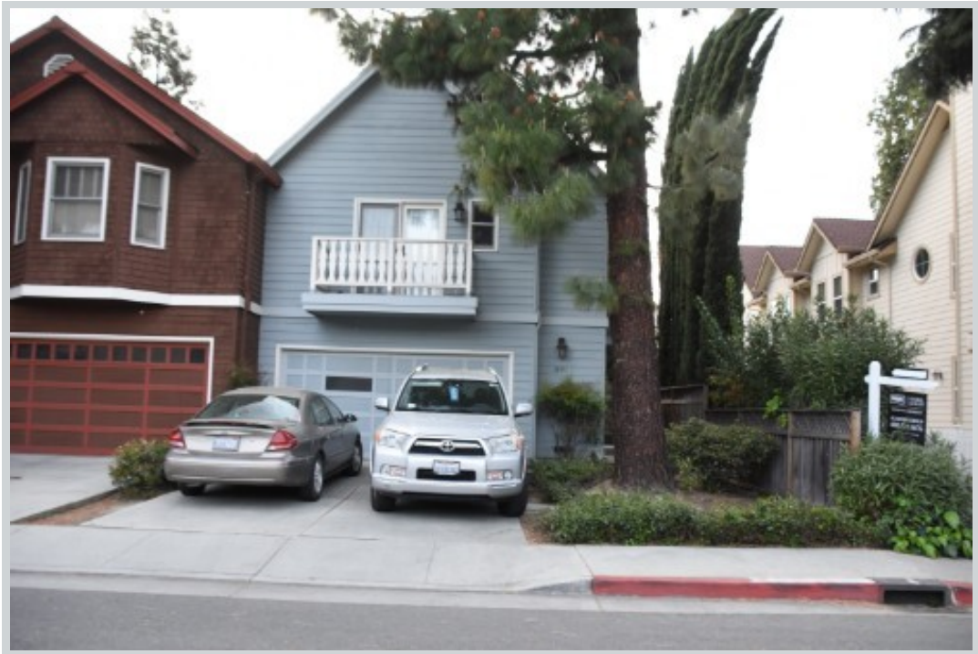
Subject 491 Boynton Ave
