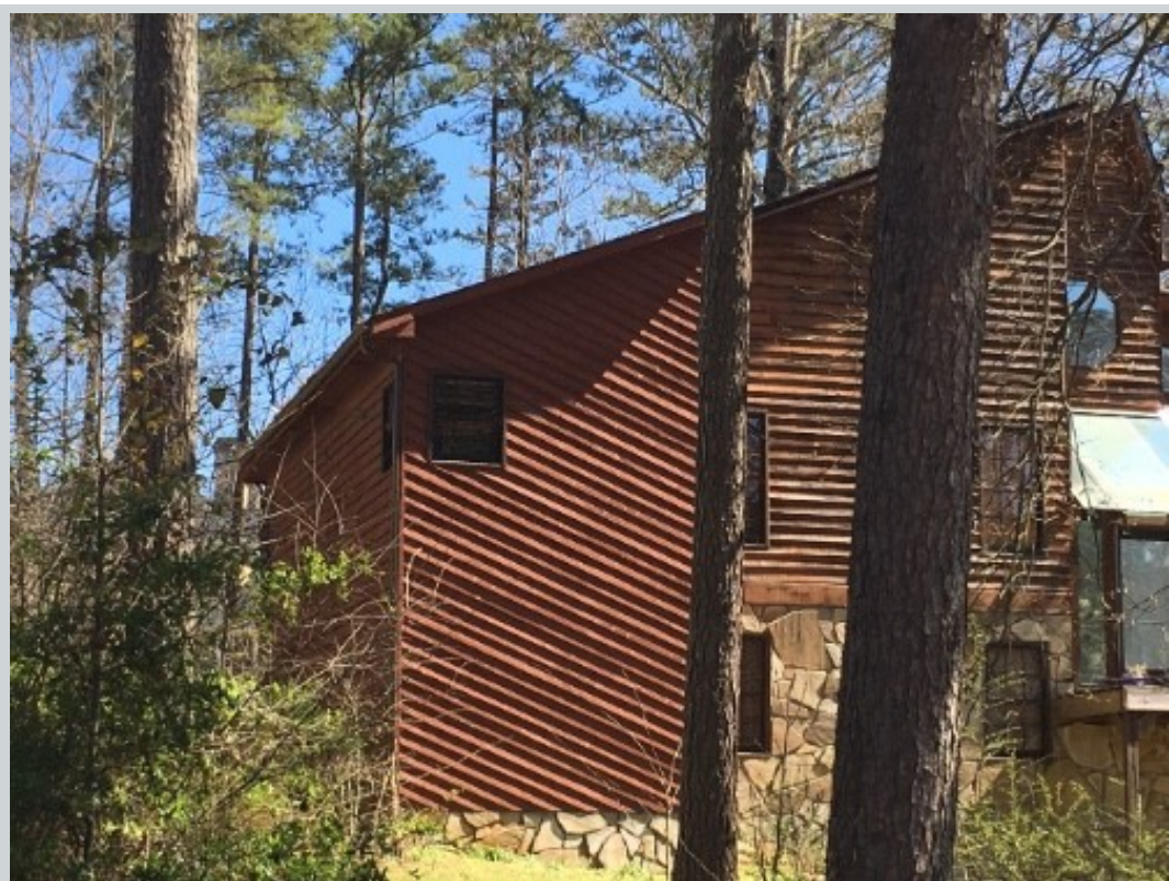
Subject 4800 Forest Way Ct Ne Comment "Damaged"
