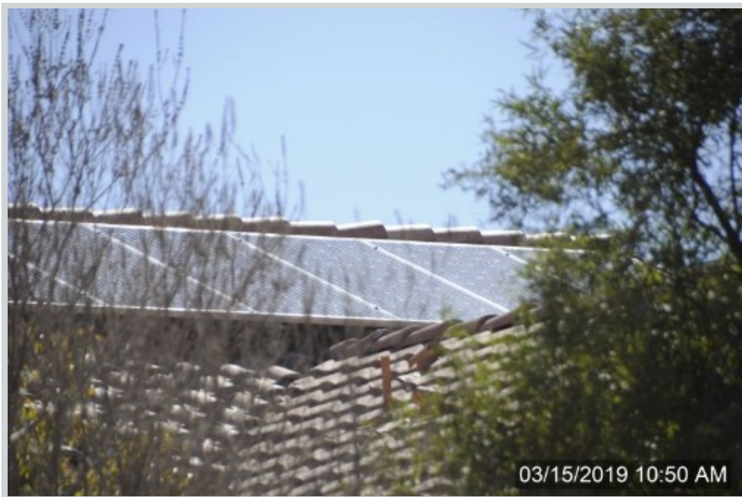
Subject 3916 Biddle St View Other Comment "Solar Panels on the Subject's Roof – Unknown Ownership, View One"
