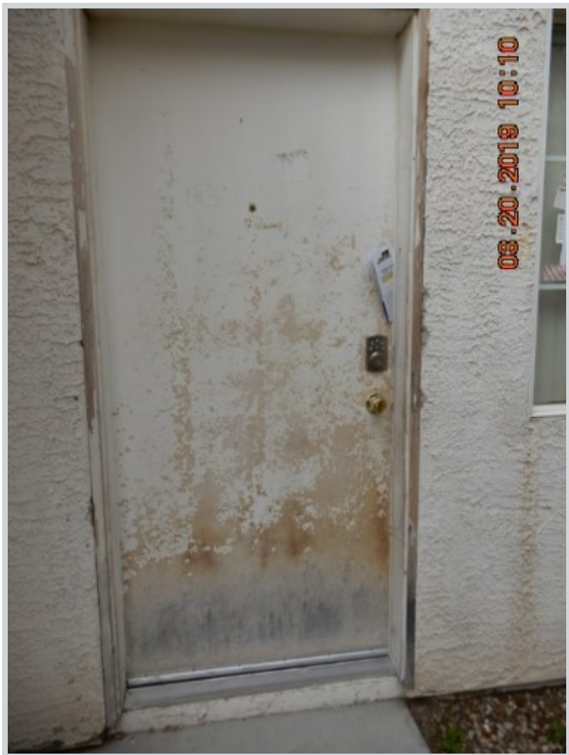
Subject 4186 Dobson Dr View Other Comment "Front door, trim and door needs paint. "
