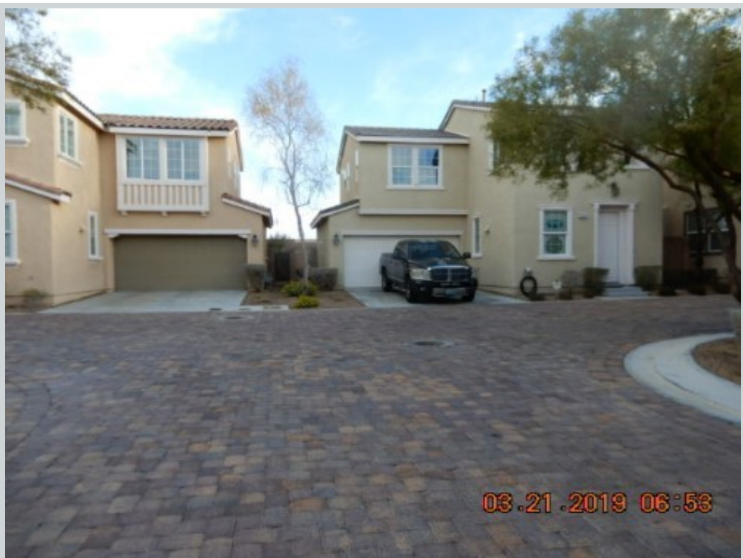
Subject 8340 Creek Canyon Ave
