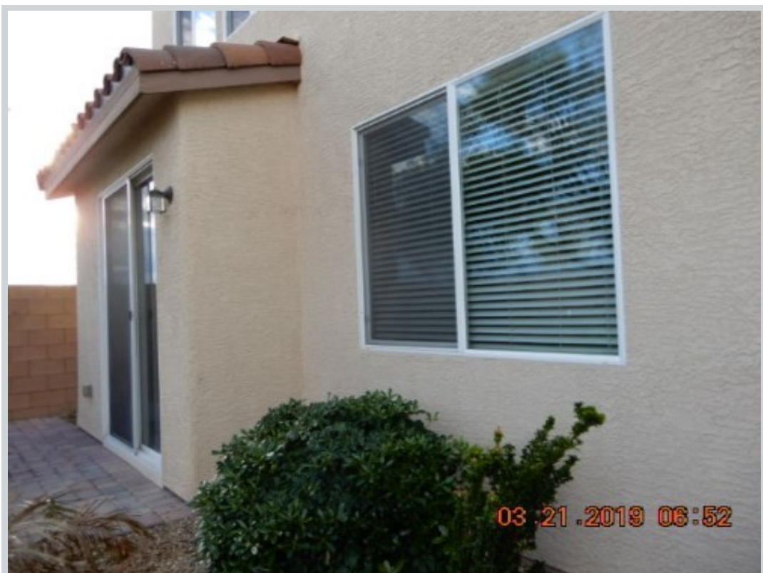
Subject 8340 Creek Canyon Ave
