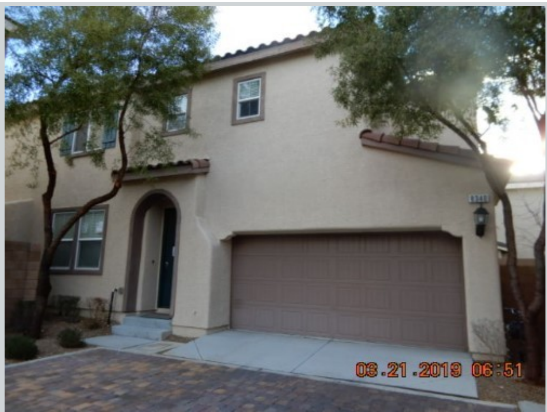
Subject 8340 Creek Canyon Ave
