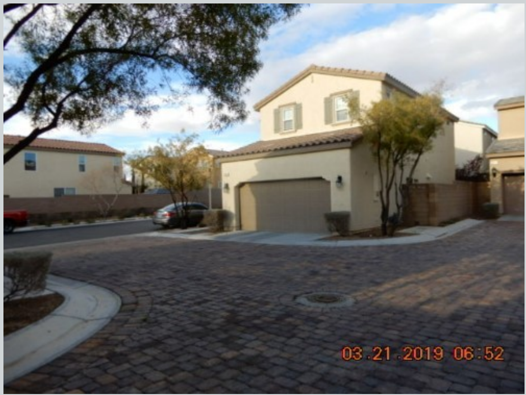
Subject 8340 Creek Canyon Ave
