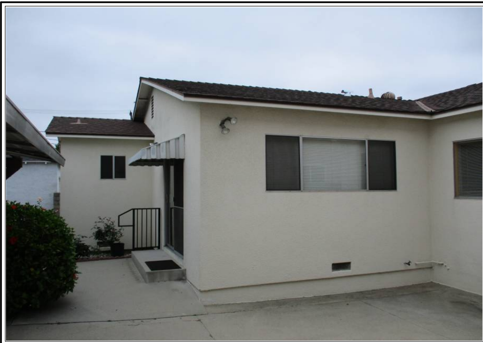
REAR OF SUBJECT PROPERTY
