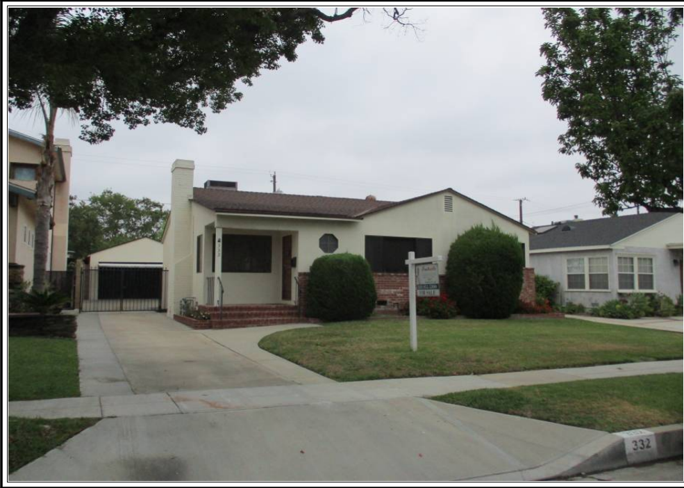
FRONT OF SUBJECT PROPERTY 332 S Virginia Ave Burbank, CA 91506
