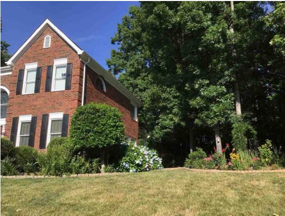
View across the street
