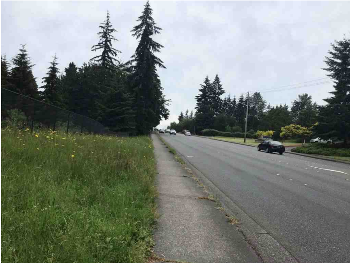
View of 108th Ave Between the subject and 108th Ave SE is a retention area (on Left)
