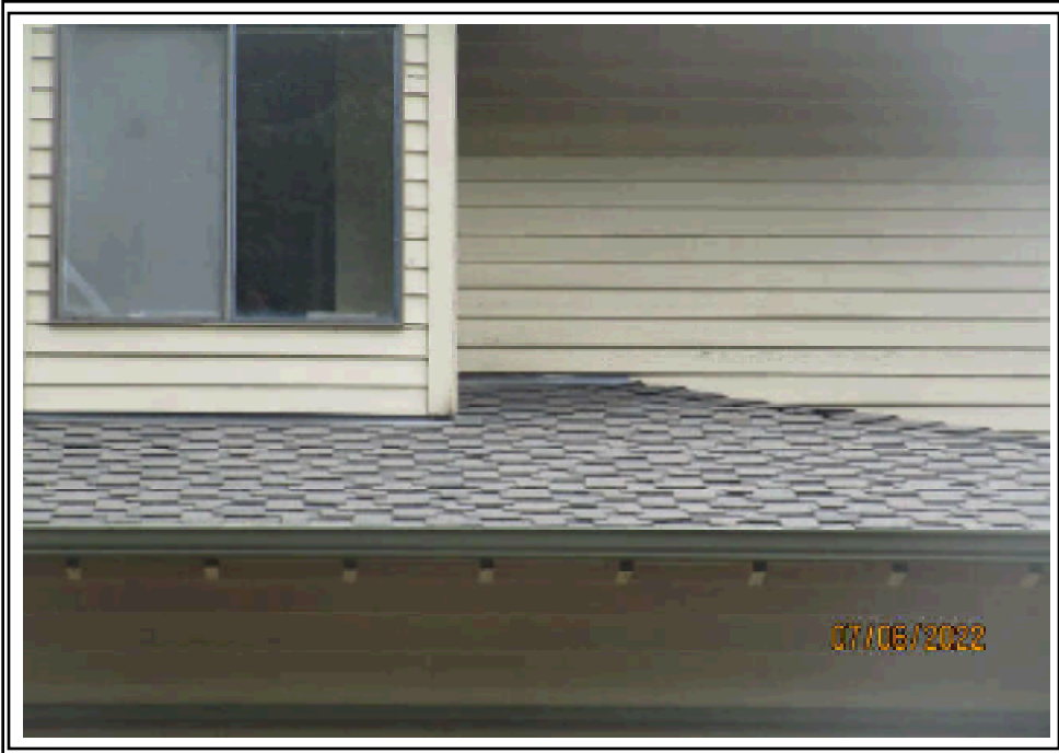
Composition roof cover appears well maintained
