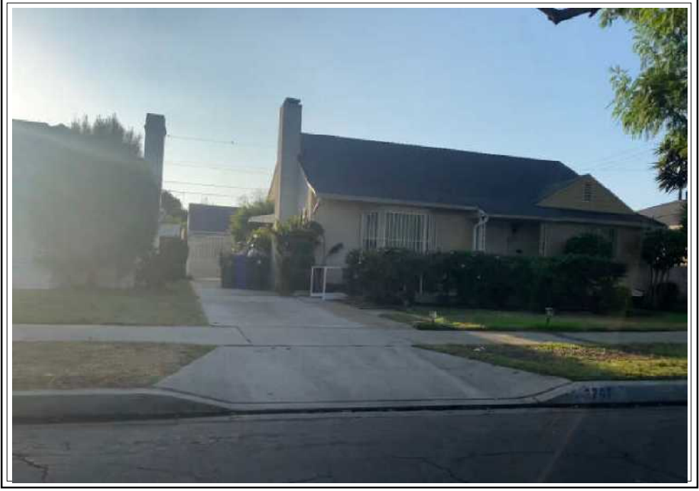
FRONT VIEW OF SUBJECT PROPERTY
