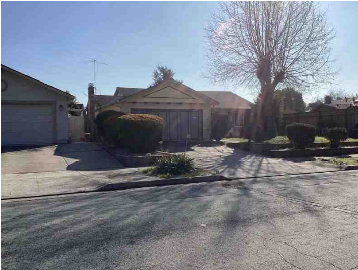
subject side (mostly front, difficult to photograph side from street)
