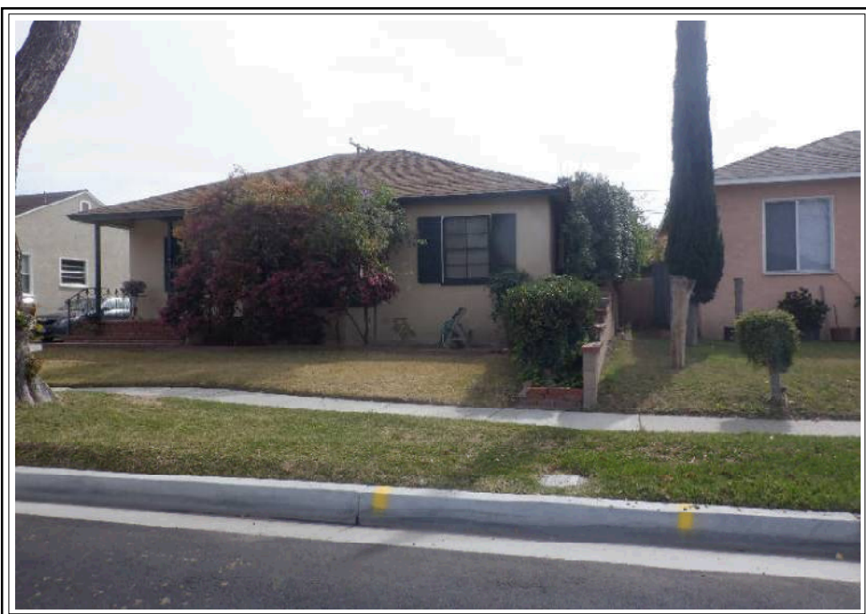
West side of subject
