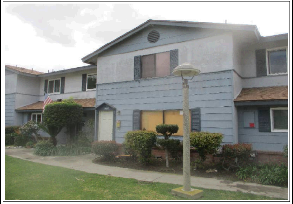
FRONT VIEW OF SUBJECT PROPERTY
