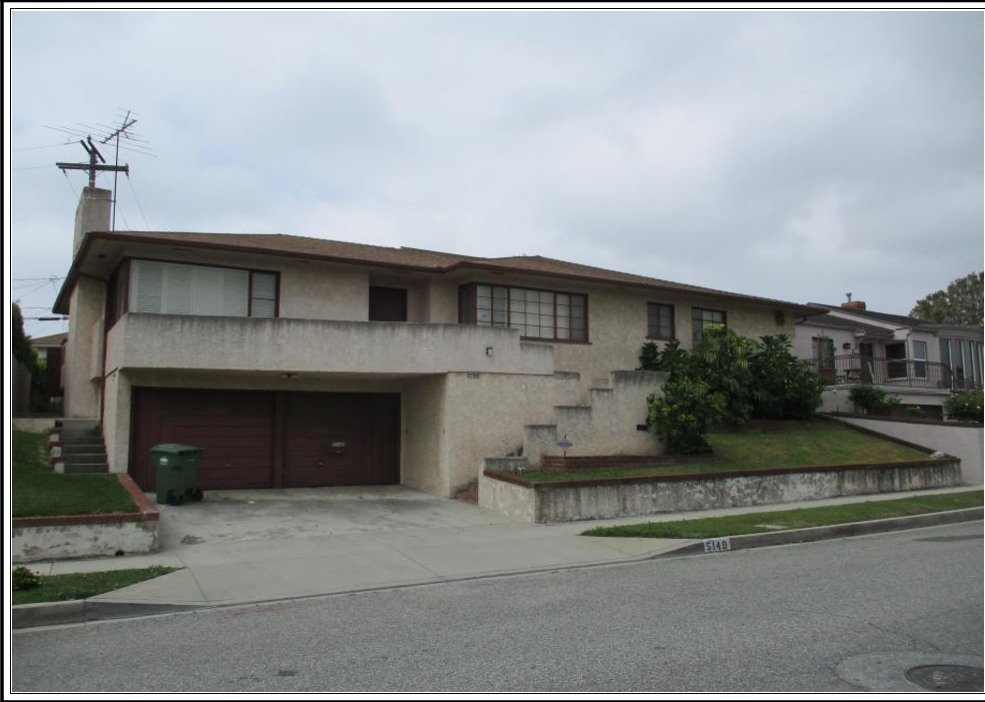
FRONT OF SUBJECT PROPERTY 5149 S Verdun Ave Los Angeles, CA 90043
