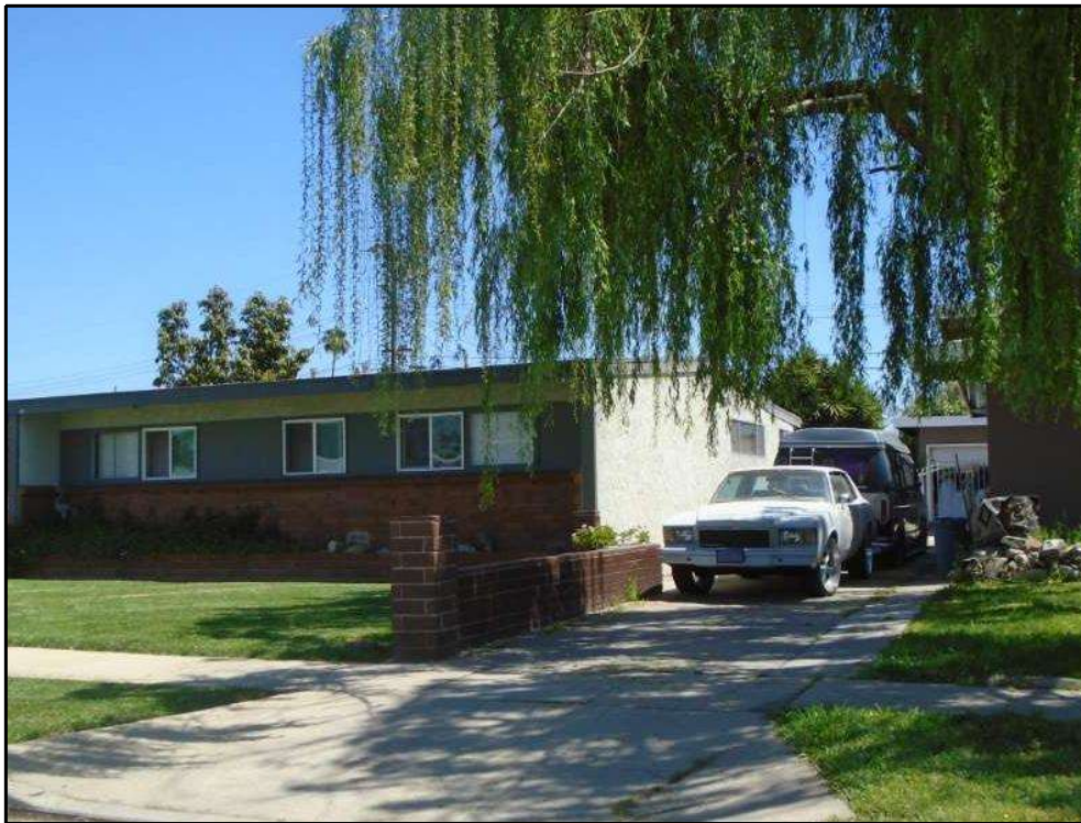
RIGHT SIDE OF SUBJECT PROPERTY
