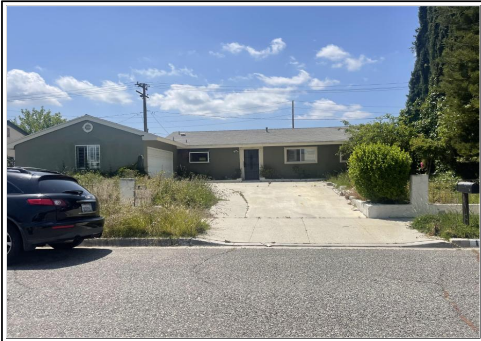
FRONT OF SUBJECT PROPERTY 1774 Hamilton St Simi Valley, CA 93065-4854
