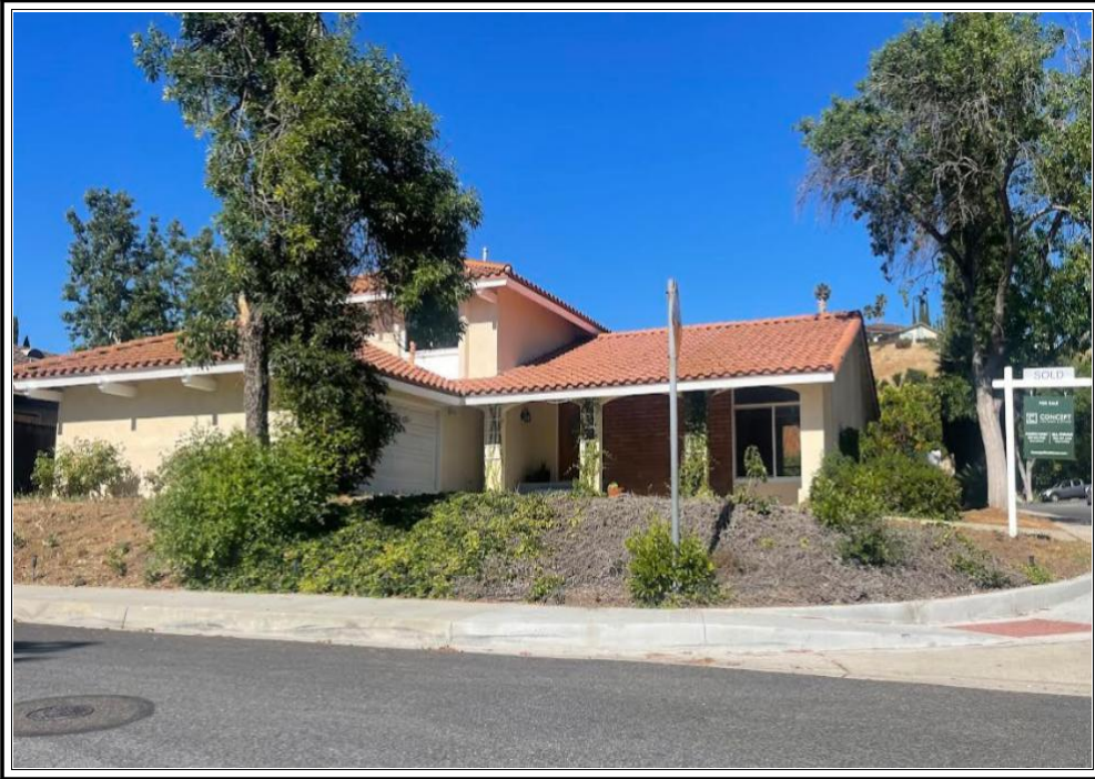
FRONT OF SUBJECT PROPERTY 1027 Stoneshead Ct Westlake Village, CA 91361
