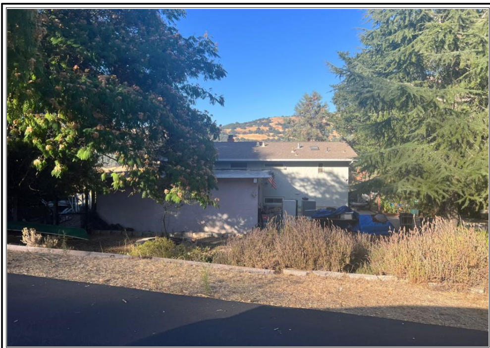
REAR OF SUBJECT PROPERTY
