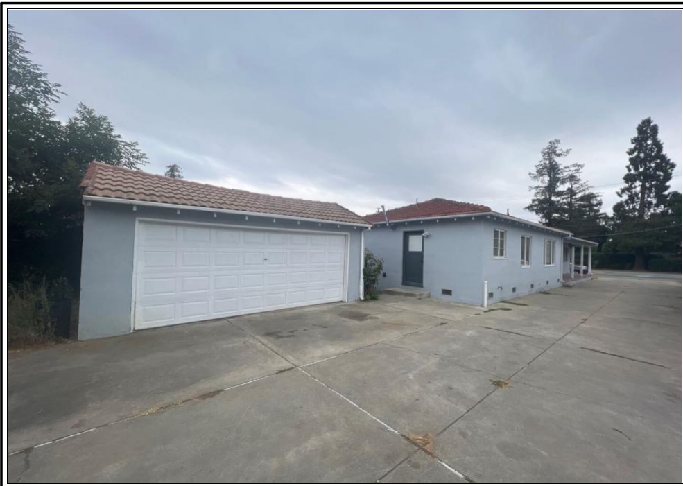
REAR OF SUBJECT PROPERTY
