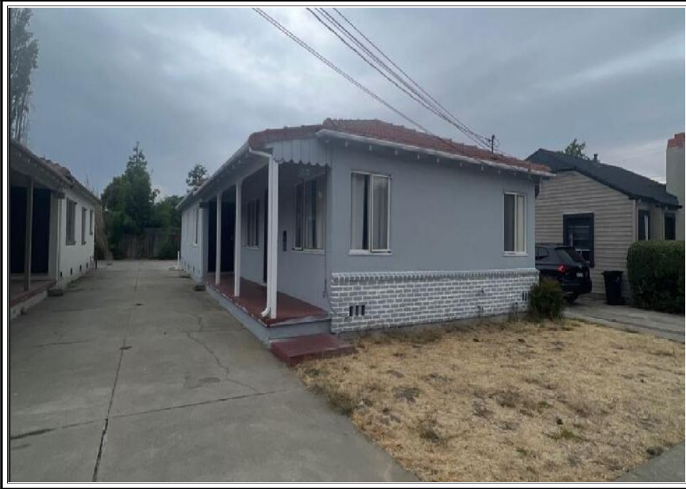
FRONT OF SUBJECT PROPERTY
