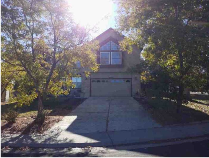
Additional Front Photo
