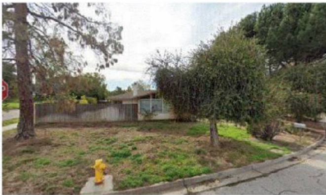
805 Via Campobello Building
