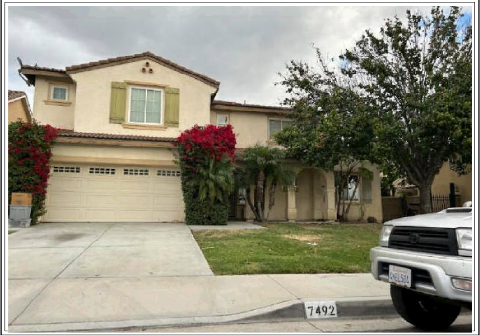
FRONT VIEW OF SUBJECT PROPERTY
