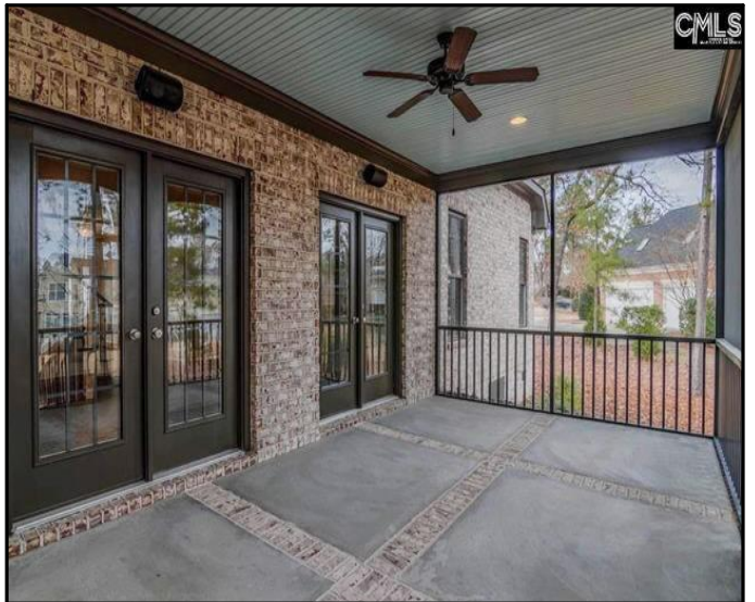
3 Redbay Court SCREEN PORCH
