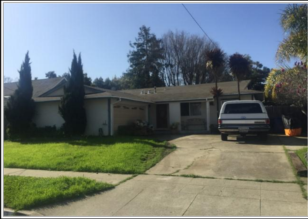
FRONT OF SUBJECT PROPERTY 6247 Montcalm Avenue Newark, CA 94560
