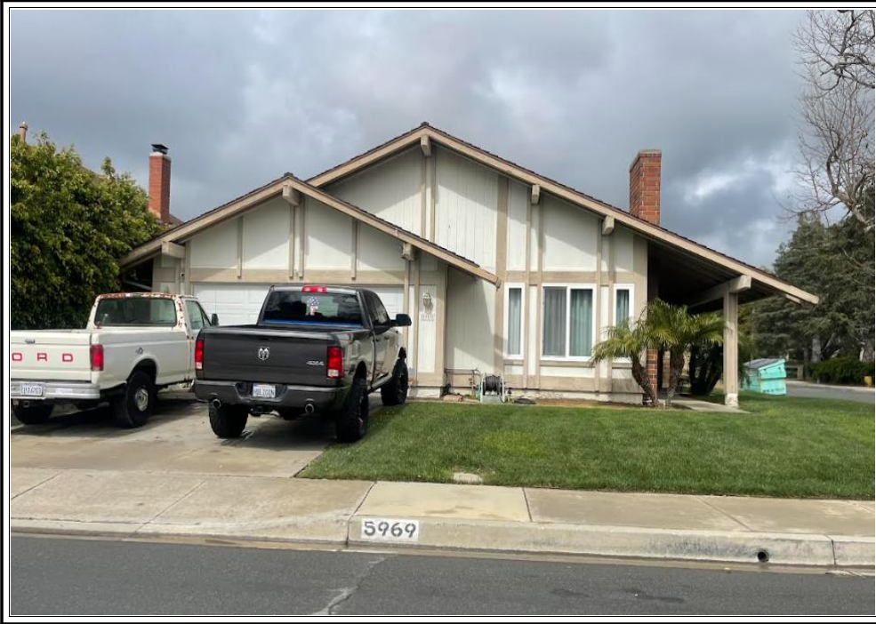
FRONT OF SUBJECT PROPERTY 5969 Joshua Trl Camarillo, CA 93012-4479
