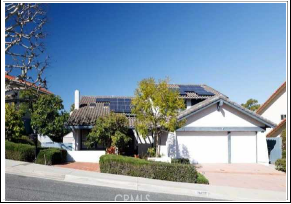
FRONT VIEW OF SUBJECT PROPERTY
