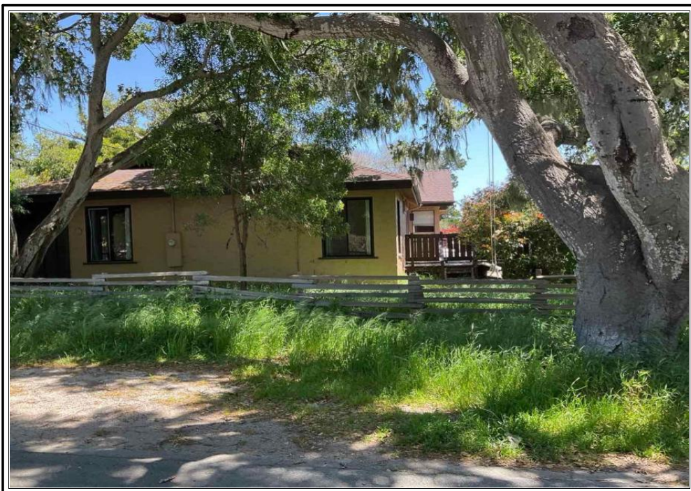
REAR OF SUBJECT PROPERTY
