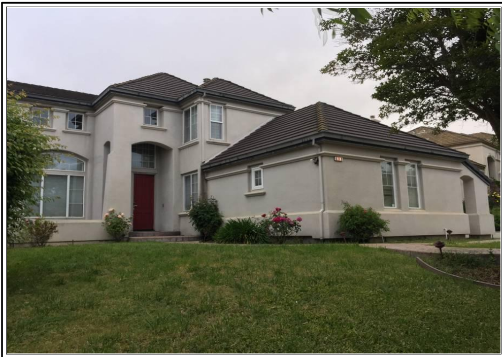
FRONT OF SUBJECT PROPERTY 553 Lower Vintners Circle Fremont, CA 94539
