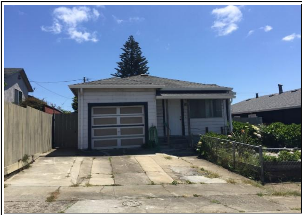
FRONT OF SUBJECT PROPERTY 124 Edison Avenue South San Francisco, CA 94080
