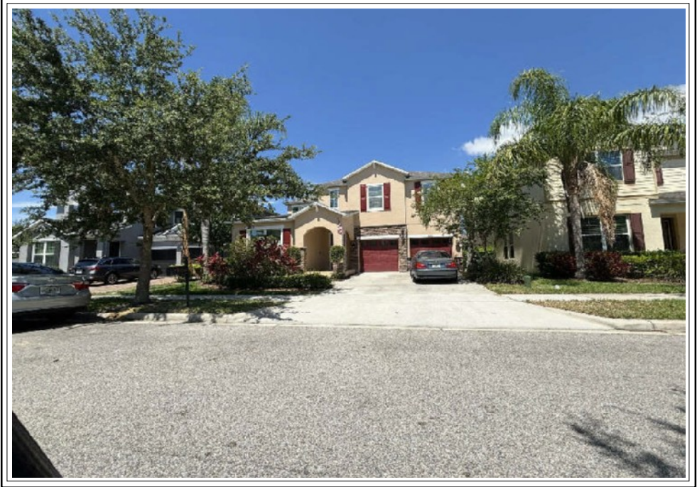
FRONT VIEW OF SUBJECT PROPERTY
