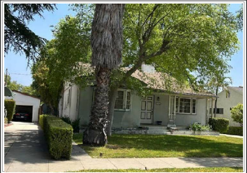
Side Subject View
