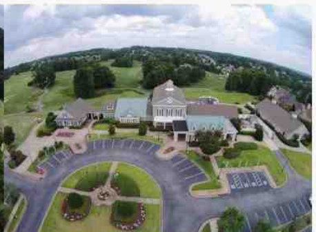
Hamilton Mill Golf Club House
