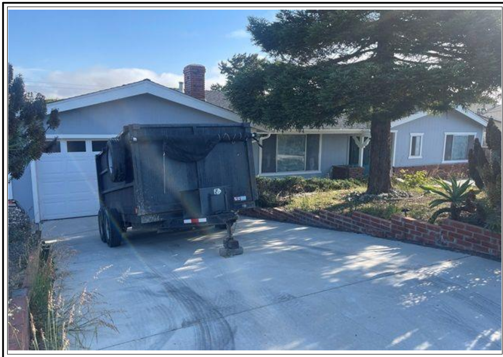
FRONT OF SUBJECT PROPERTY 716 Manzanita Drive Los Osos, CA 93402
