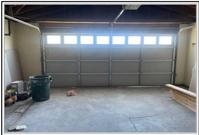
Interior of Garage
