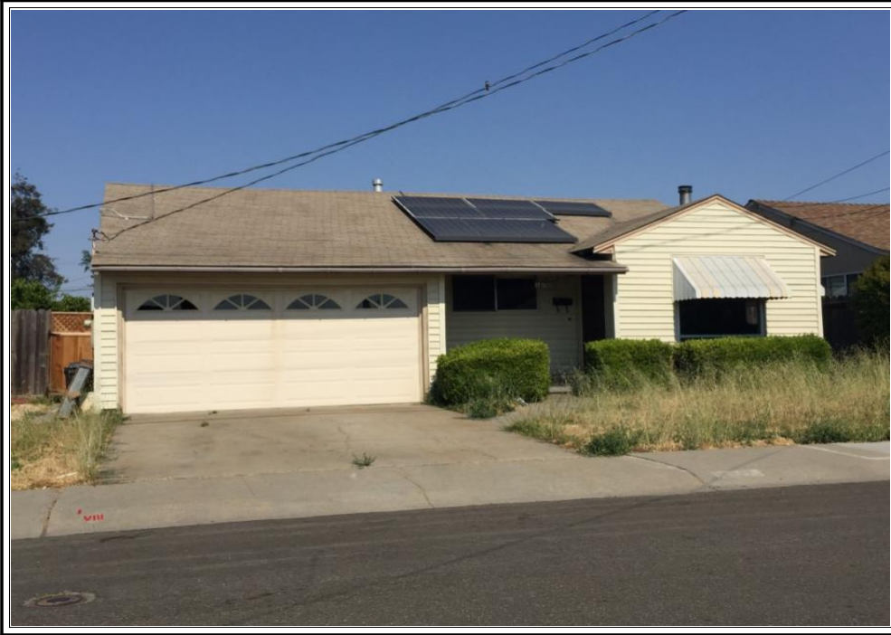
FRONT OF SUBJECT PROPERTY 14700 Acacia Street San Leandro, CA 94579
