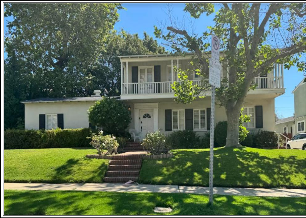
FRONT OF SUBJECT PROPERTY 1244 Woodruff Ave Los Angeles, CA 90024-5128
