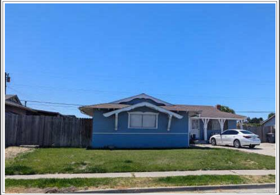
FRONT VIEW OF SUBJECT PROPERTY
