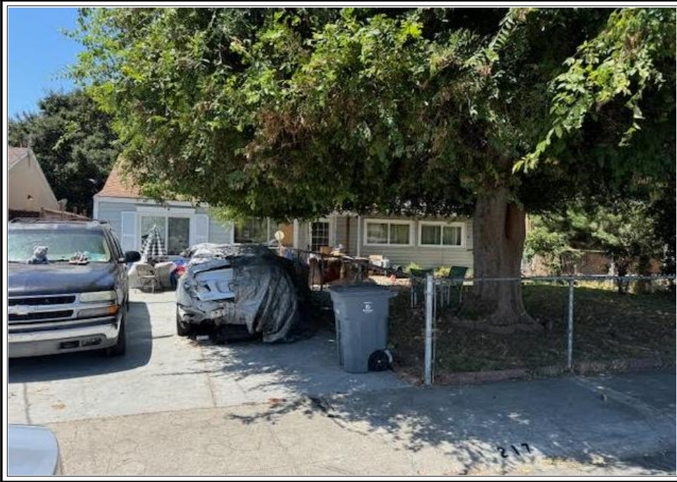
FRONT OF SUBJECT PROPERTY 217 N CRAGMONT AVE SAN JOSE, CA 95127
