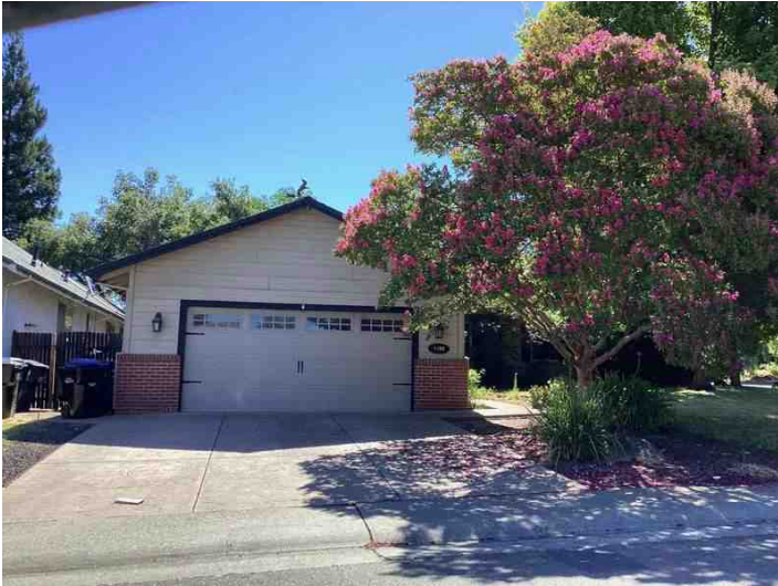
Garage and Driveway
