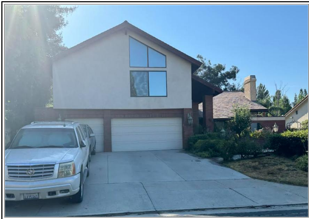
FRONT OF SUBJECT PROPERTY 11048 Oso Ave Chatsworth, CA 91311
