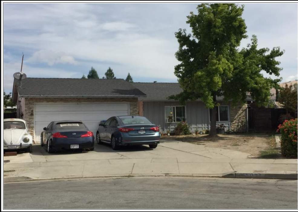
FRONT OF SUBJECT PROPERTY 2034 Cove Court San Jose, CA 95148
