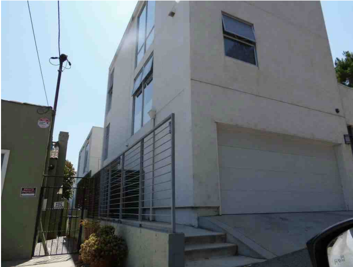
REAR OF COMPLEX
