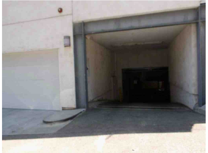
ENTRY TO BASEMENT GARAGE
