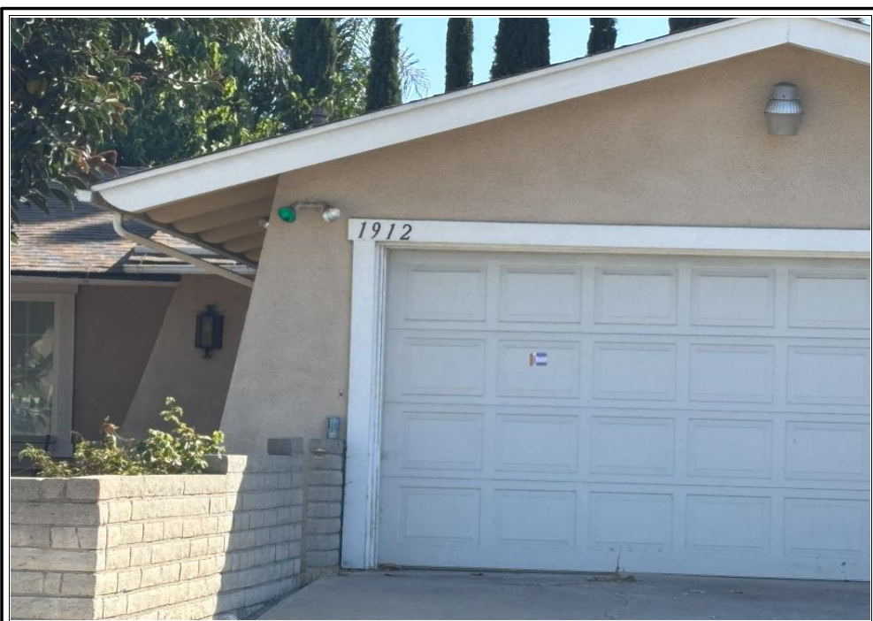
Alternate Front View of Subject with Address
